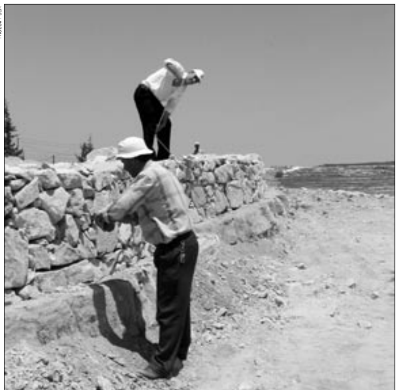
Workers build a retaining wall in Halhoul.
