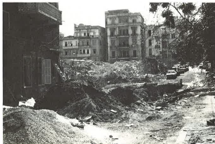
Reconstruction of sewage pipes begins in Beirut
