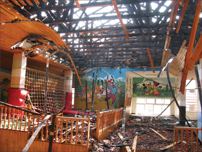
The children's ward in Al Quds Hospital was destroyed.
