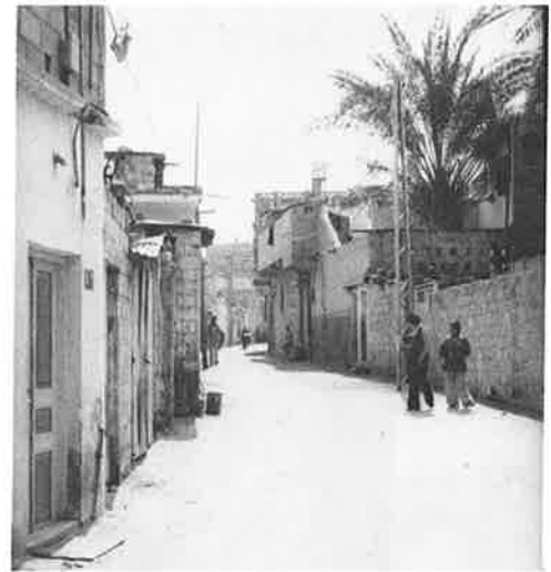
Water pipes from ANERA were used for new sewers in poor neighborhoods in Gaza.
