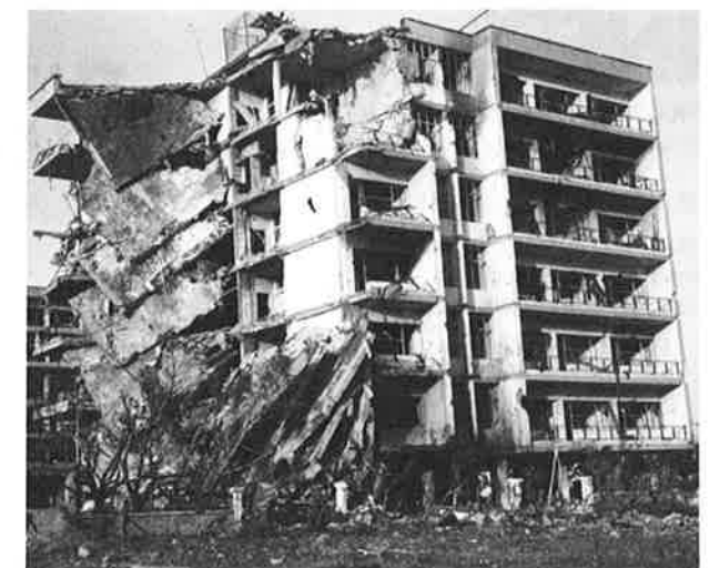
Modern buildings damaged in the Civil War still await reconstruction.
