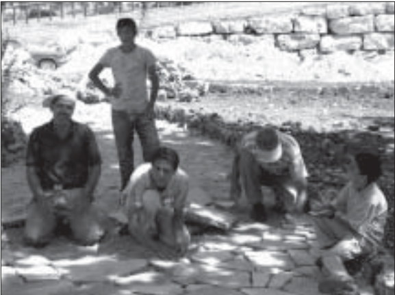
JOB CREATION PROGRAM - QABALANI, WEST BANK/WASER, QADOUS
