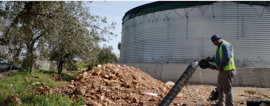
This tank collects the cleaned wastewater. Distribution pipes are being attached.
