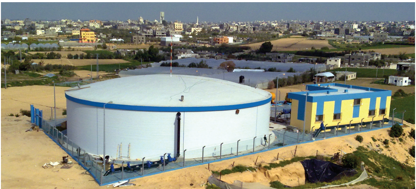
Anera built this reservoir in Khan Younis, Gaza. It is a clean and reliable source of water for 70,000 people.
