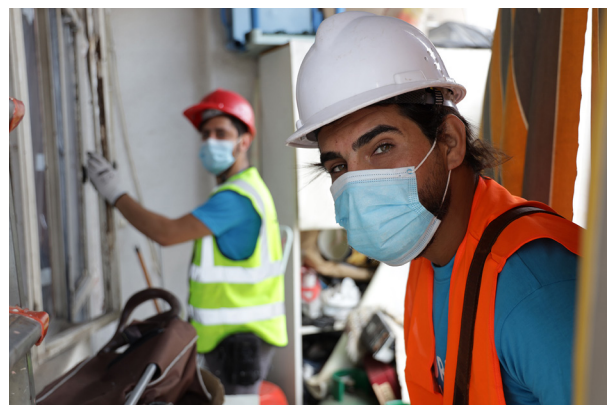
Anera construction vocational students renovate a home damaged in the 2020 Beirut explosion. Students gain job skills training while earning an income for their work.
